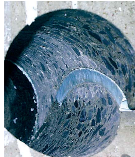
Injected construction joint
