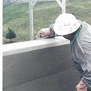
Working in Zentrifix F 92 with a hard rubber float.
