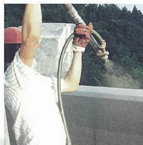
Spraying on the coating
