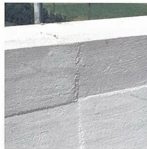
Finished scratch-coat
