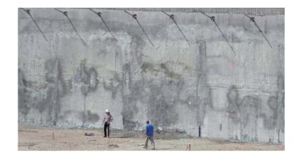
The objective of the injection and local conditions determine the individual technical application in each case. Depending on the problem, packers are positioned alongside the areas that need waterproofing and reinforcing and injections are carried out.
