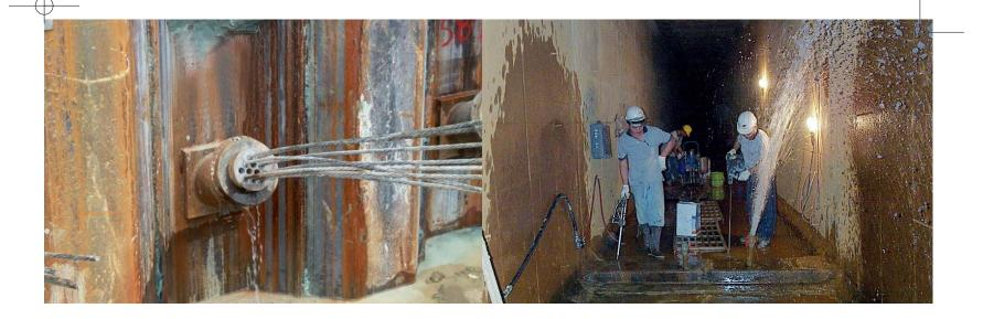
The waterproofing and reinforcing injection of supporting subsoil ensures smooth building construction and creates security for the new structure. Preventative injections, such as waterproofing in transition areas of HDI-walls, sheet pile walls
